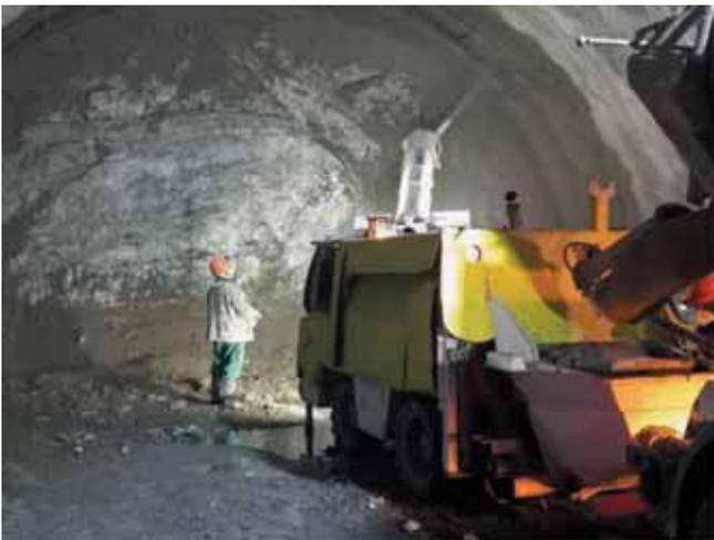
Рис. 9. Установка сталеполимерных анкеров  $l = 2,0$  м
