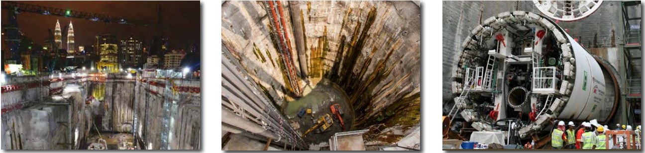
TRX Station and TBM Machines
