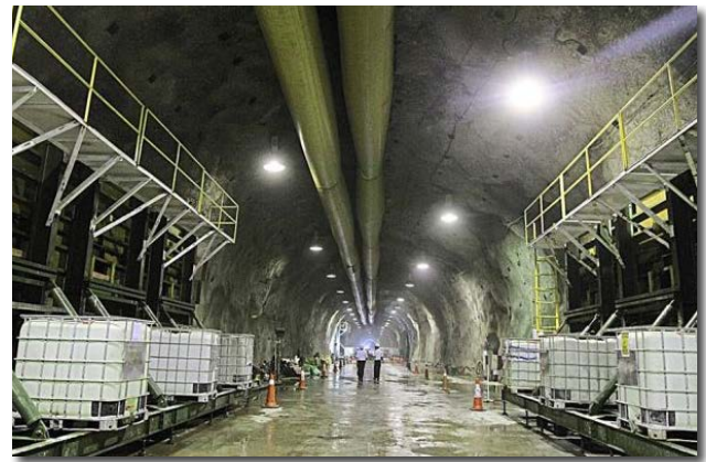
Sungai Selangor Water Transfer Tunnel
