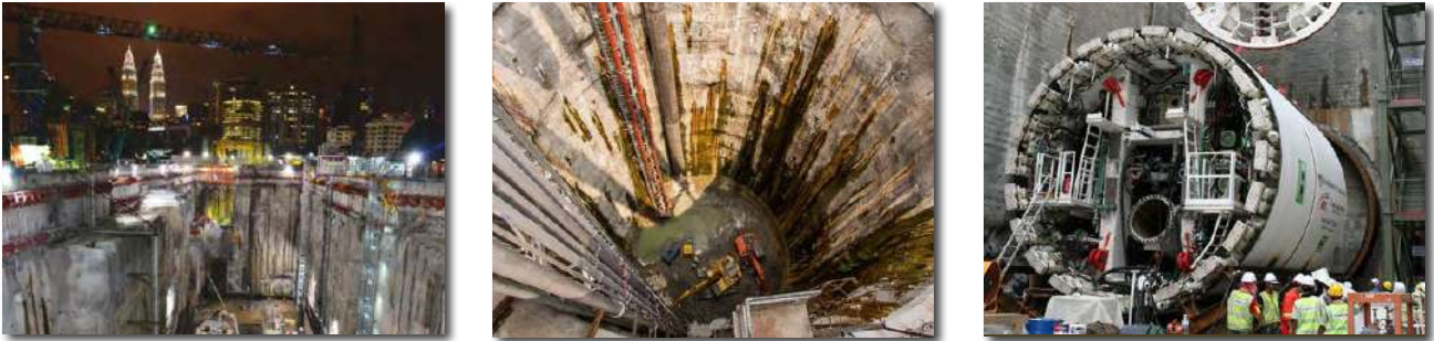
TRX Station and TBM Machines
