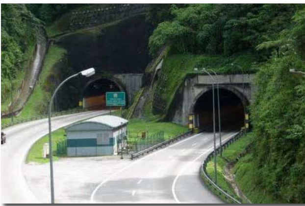
Karak Highway Twin Tunnel
